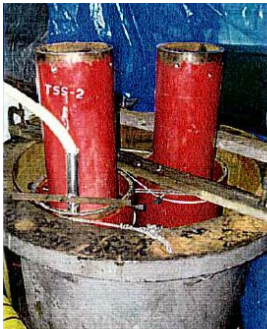
Pouring of non-conducting shear bulkheads
